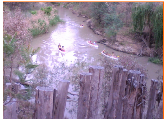
Photo Above: The foreground shows bank stabilisation techniques along the Broken River.
